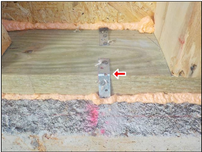
Example, missing nails
