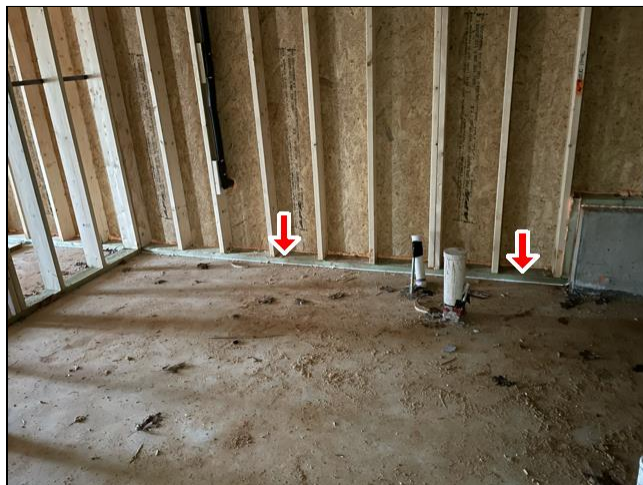
Missing anchors bathroom area
