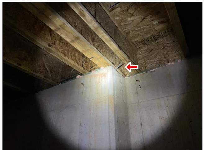
Loose strap front wall below front porch
