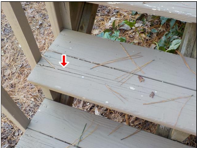
Example, cracks step
