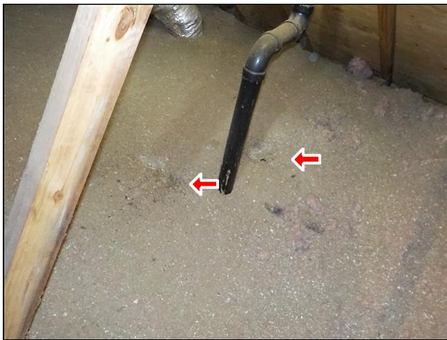
Evidence of previous wetness on insulation
