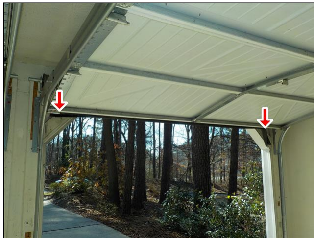
Sensors installed improperly
